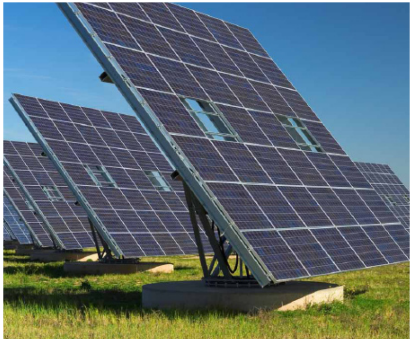
Figure 4.3 | Solar panels vary in form and scale. The smaller rectangular panels have a height of 4m, while the larger disk shaped panels reach a height of 14m.
