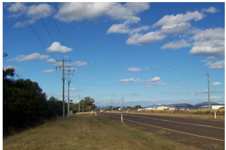
Figure 4.5c | Nearly all routes considered for transmission line options support existing power lines that will be amalgamated into the new transmission line structures.
