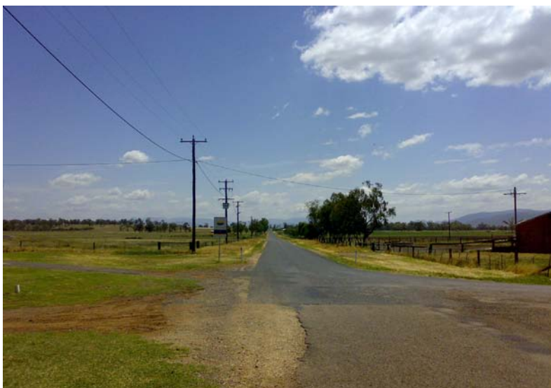
Figure 4.5d | Options 3 and 4, in small part, follow Back Muswellbrook Road. This road currently supports a distribution powerline, the cables of which would be incorporated into the new pole structure.
