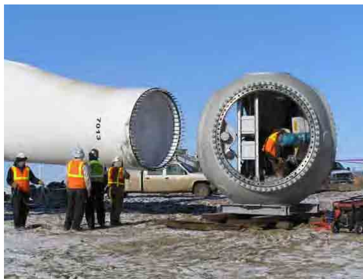
Crane crews putting together a Turbine Rotor Assembly
