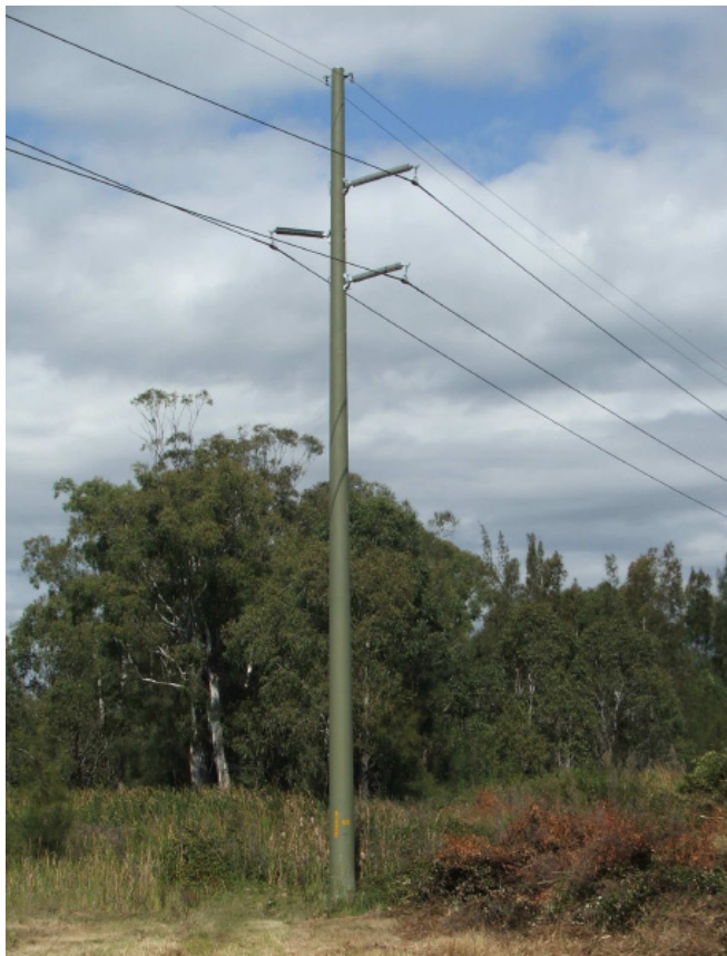
Figure 19.11 Typical Concrete Pole Configuration (Energy Australia 2008)
