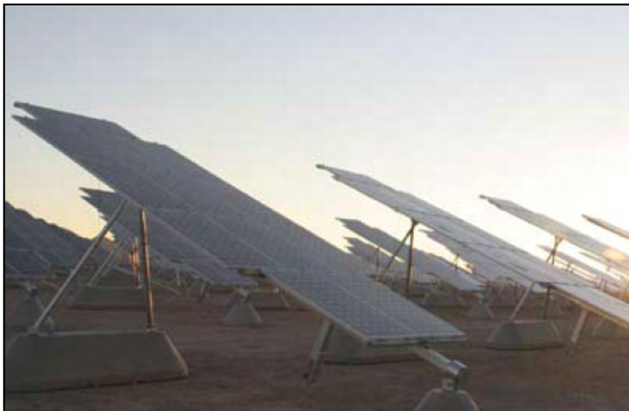
Figure 2.7 – Solar PV Single Axis Power Tracker Supporting Structure (Example)
