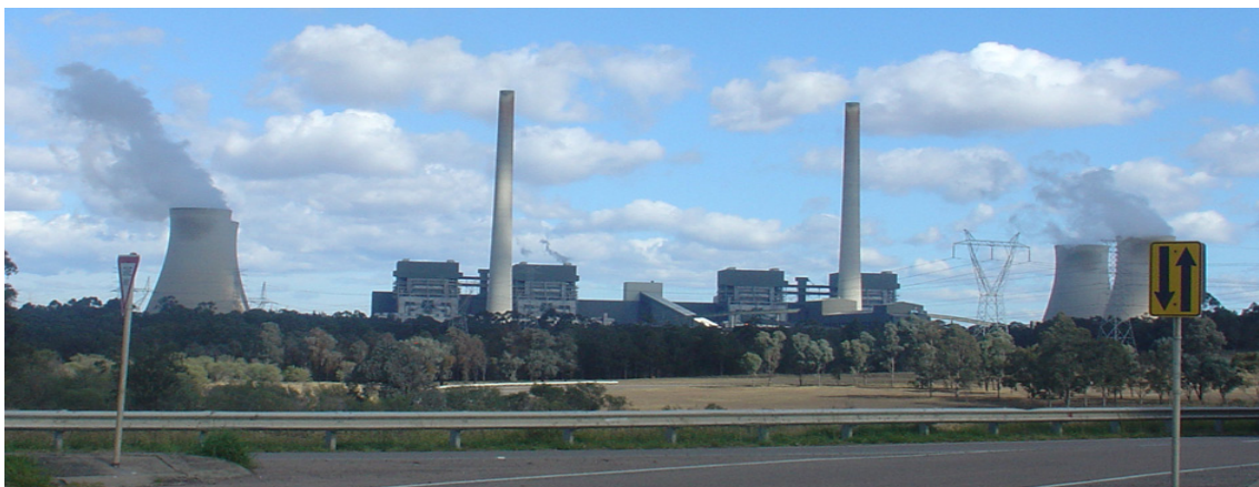
Figure 6.7 Ravenswater Coal-fired Power Station
