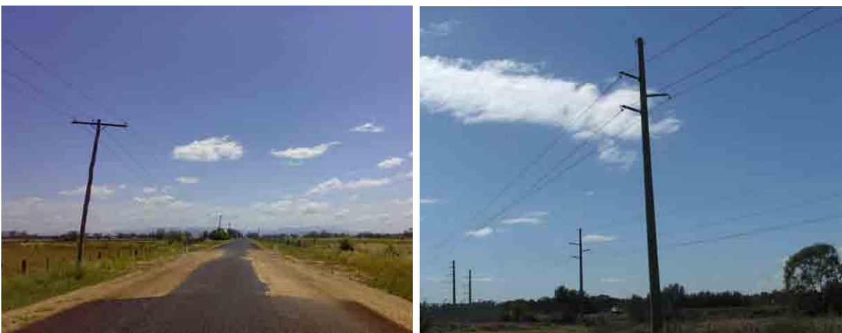
Figure 19.6 Photographs showing existing timber poles (left) and proposed replacement concrete poles (right) (Energy Australia 2007)
