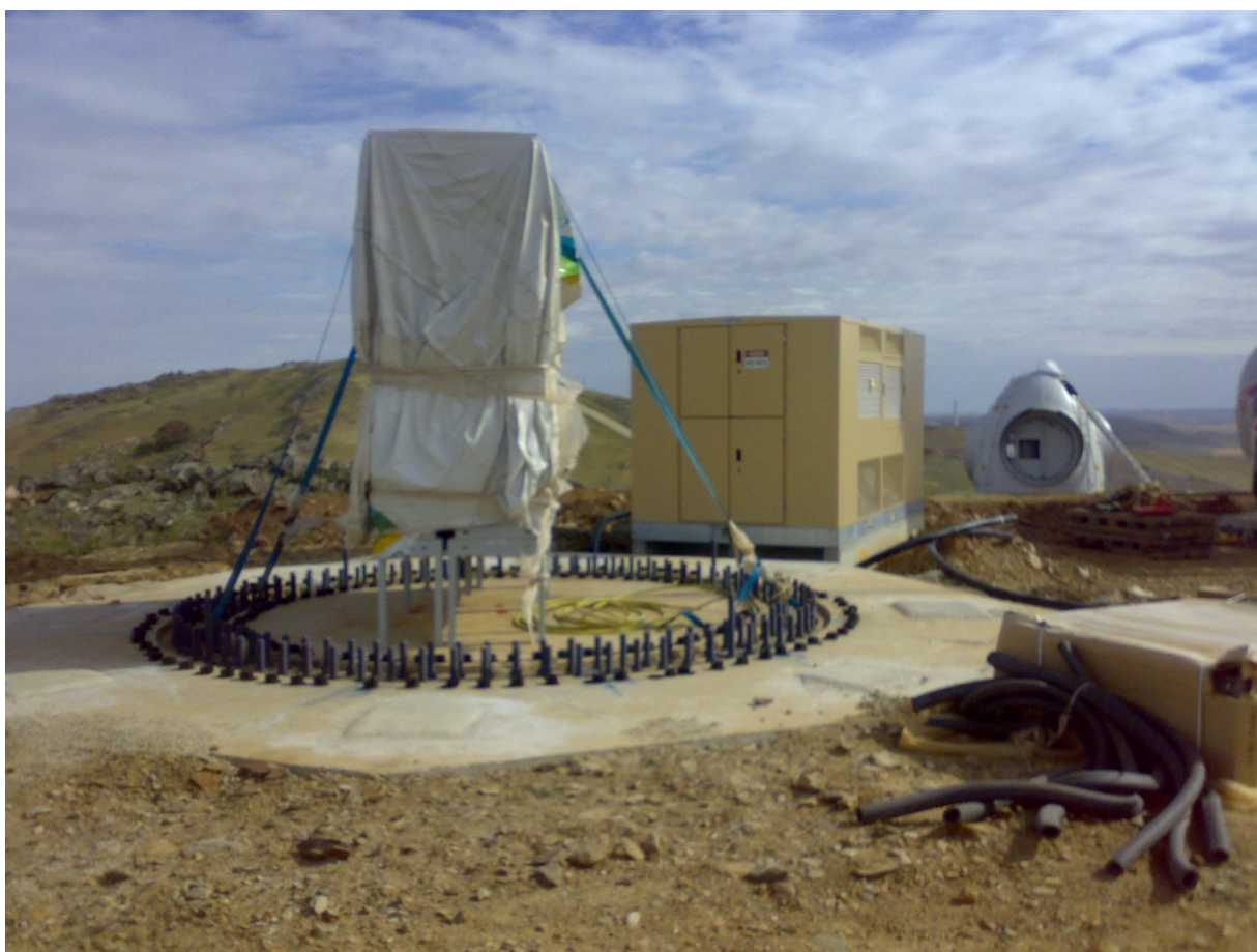
Figure 3.3 Typical Concrete Wind Turbine Foundation
