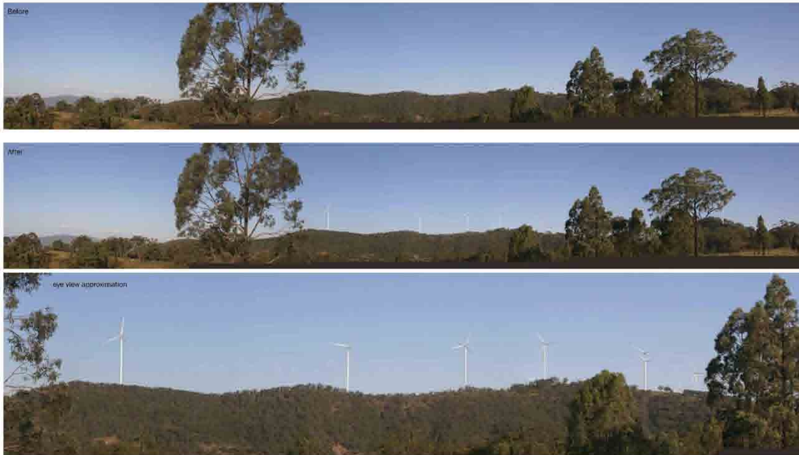
Figure 6.16 | View from Clifton Gardens on to the western side of Mountain Station from approximately 1.5km away.
