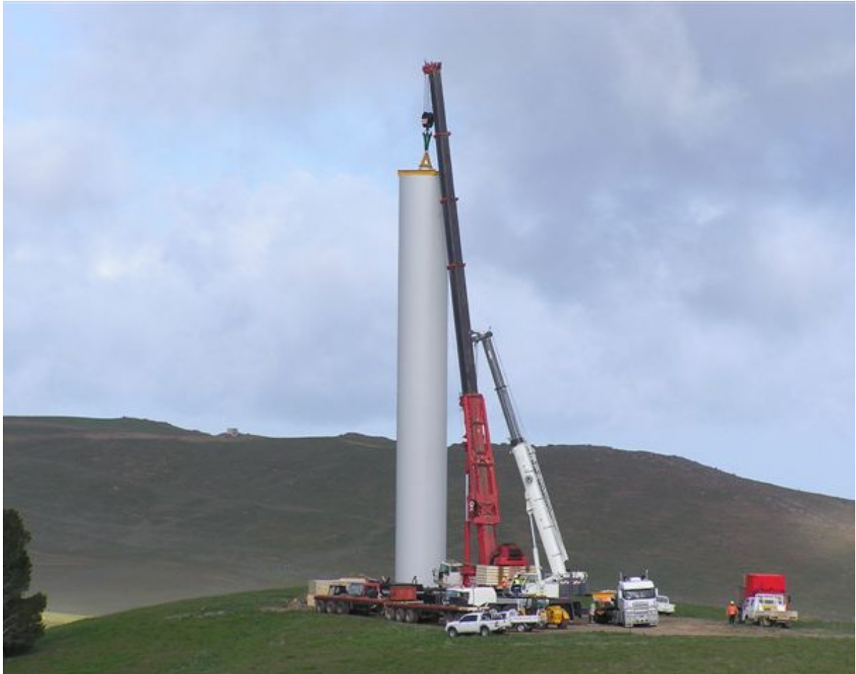
Figure 3.5 Crane Erection of Tower Tube.
