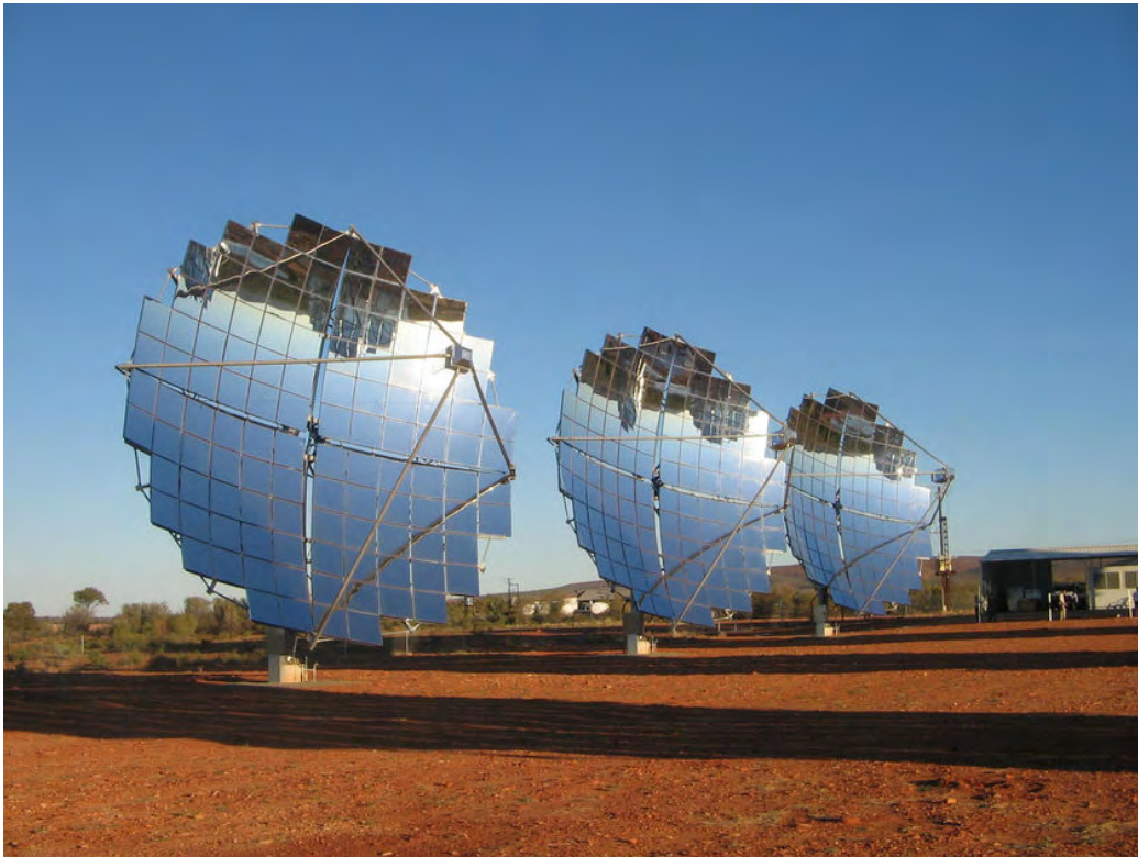
Figure 2.9 – Example of a Photovoltaic Concentrator Structure (PVC) (Courtesy of Solar Systems Australia)
